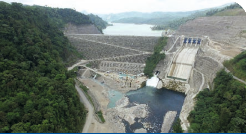
Costa Rican Reventazon hydroelectric dam (305 MW) is the second biggest infrastructure project in Central America after the Panama Canal and the largest of its kind in the region. This dam is a living example of the lies propagated by the Oxford Said Business School economists about dams: The cost of the project by the Instituto Costarricense de Electricidad (ICE), the State power company, came at only US$1.4 billion dollars and it was completed three months ahead of schedule.
