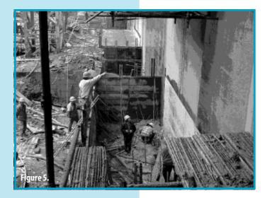
Figure 5. Construction of concrete blocks at the heel of the dam below low level cracks. repair system. The thickness of the slab is 40cm below El. 45m, and 25cm above El. 50m. In the inverse slope areas between elevations 45m to 50m, the surface of SR2 cover plate is protected by a PVC cover with 2cm thickness. For #5 to #17 spillway dam sections below El. 30m, the concrete slab is placed to protect the SR2 cover plate.
