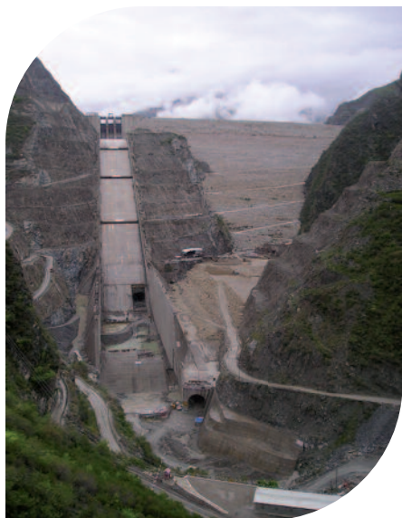
(3) Tehri Dam in India
