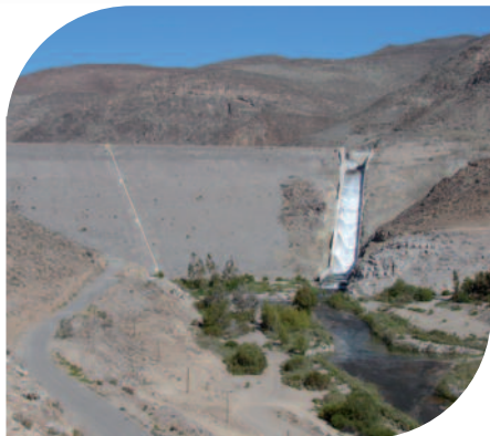
(2) Santa Juana Dam in Chile
