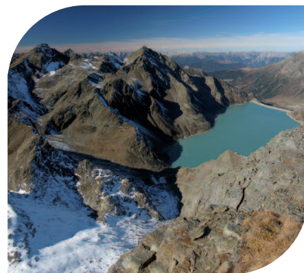
(1) Finstertal Dam in Austria
