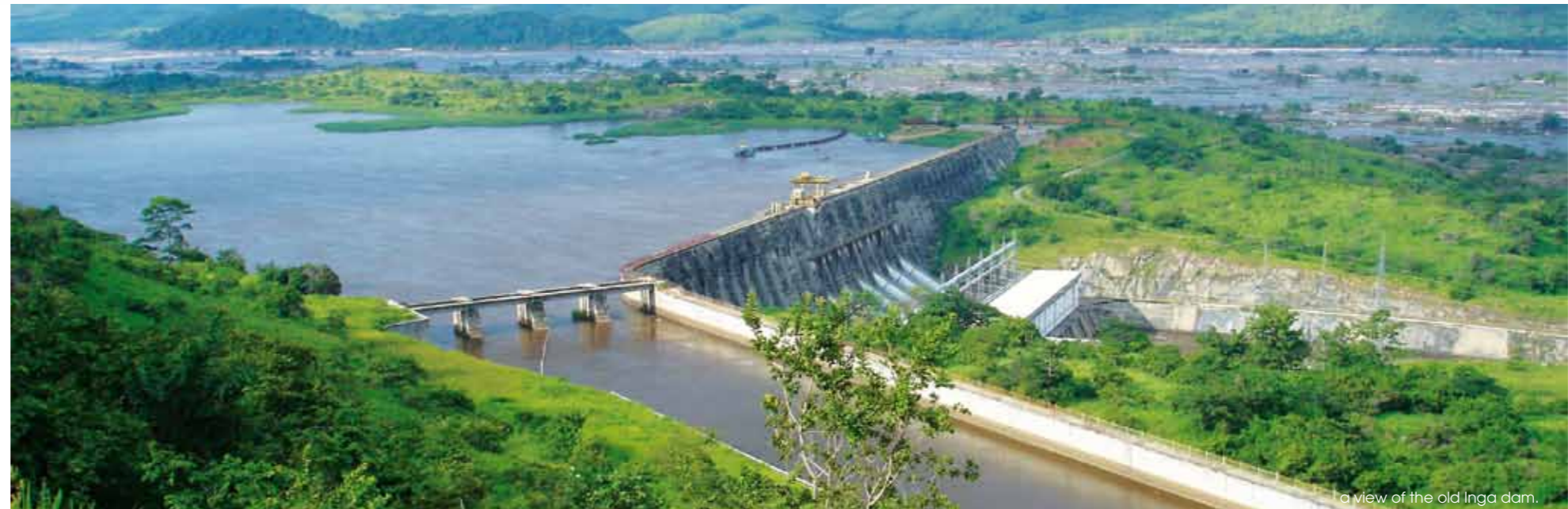
a view of the old Inga dam.
