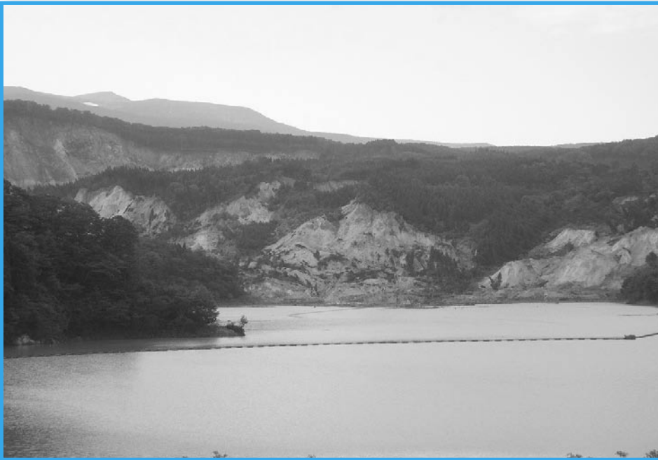
Photo-2 The slide mass at Aratozawa Dam
