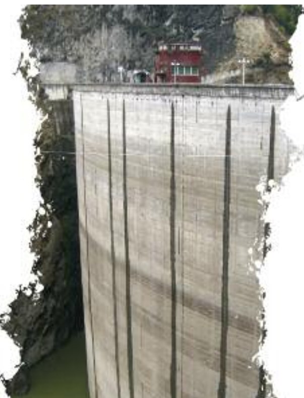
Fig. 1: Upstream face of Shapai RCC arch dam
