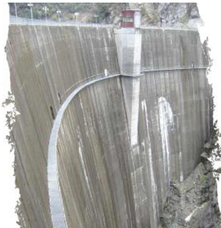
Fig. 2: Downstream face of Shapai RCC arch dam
